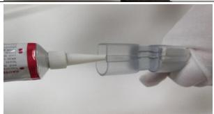
3. Using silicone sealant glue, seal the both ends of straight connector
